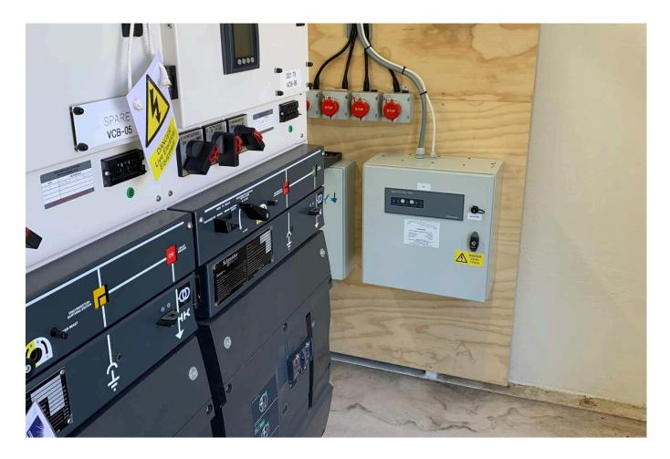
Figure 4-6 - SynchroTeq Retrofit Installation
