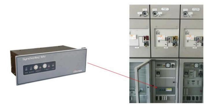
Figure 4-10 - SynchroTeq Installed within Switchgear
