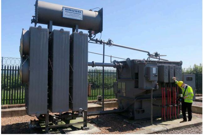
Figure 4-9 - SSEN 15MVA transformer
